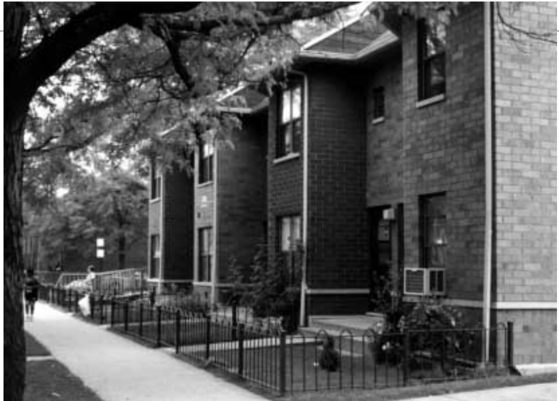
At West Town Housing Partners, five clusters of well-maintained townhouses are scattered throughout the West Town and Logan Square communities of Chicago. Satisfied tenants mean the wait list opens only once every three to four years. Photo courtesy of Bickerdike Redevelopment Corporation.
