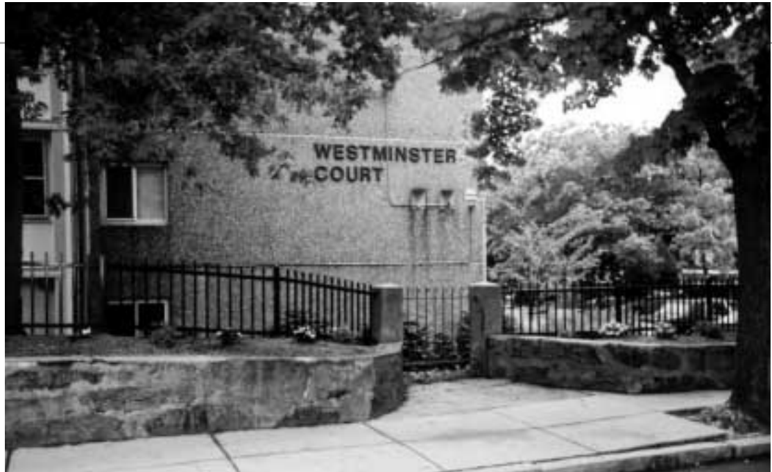
Built in the late 1960s and rehabilitated in 1995, Westminster Court Apartments is comprised of three, three-story buildings clustered around a large courtyard. Photo courtesy Urban Edge.
