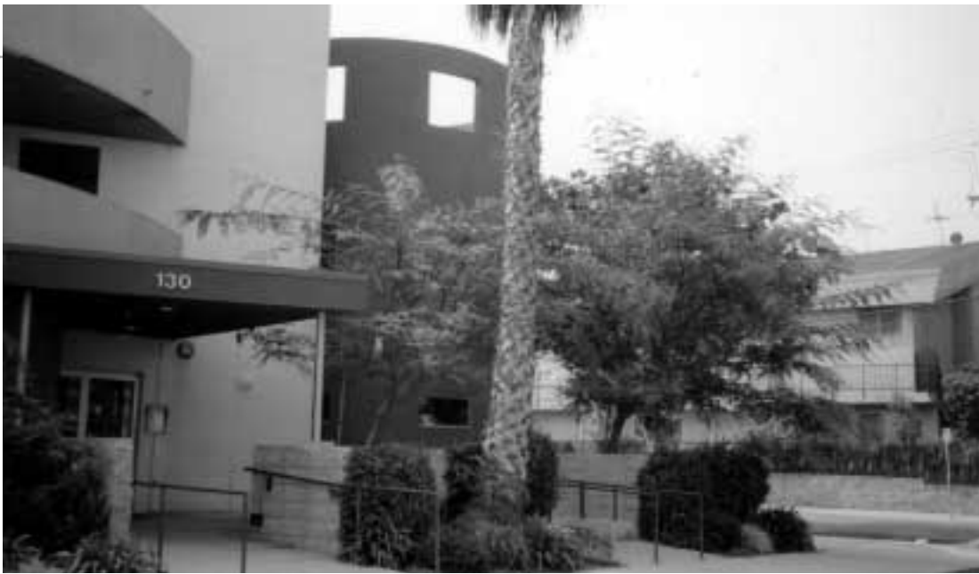
Vista Nueva Apartments is distinguished by its striking architecture, which integrates well into the surrounding Los Angeles neighborhood. Photo courtesy of A Community of Friends.
